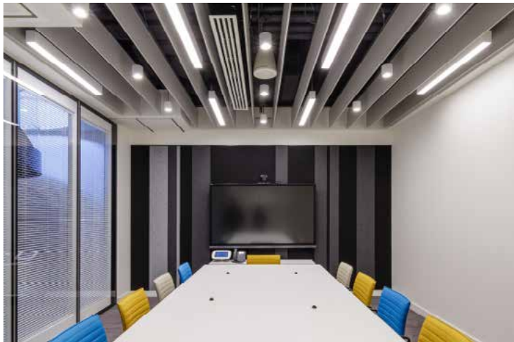
As with wall panels, Baffles and Rafts act as an effective sound absorber, helping to eliminate unwanted noise within the space.
